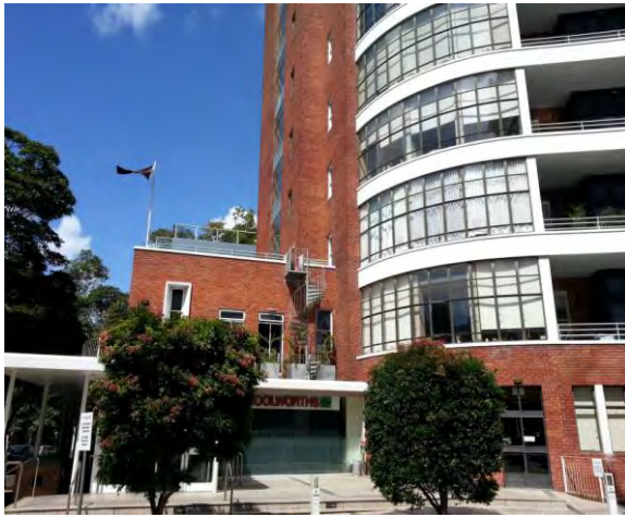
FIGURE 1. NON TRADITIONAL SUPERMARKET FORMATS
